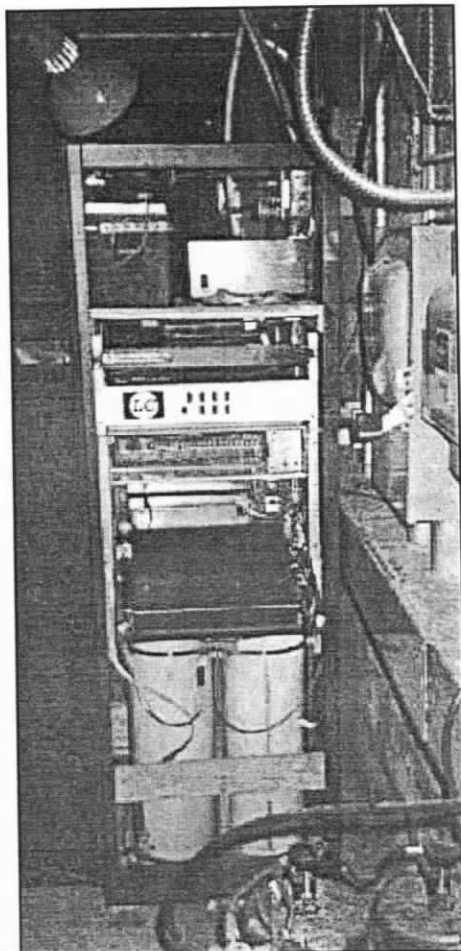
The 146.94 repeater with doors removed. Backup battery and power supply are visible on the top shelf. LC Controller, modem, and radio gear are in the center. Duplexers can be seen at the bottom of cabinet.
